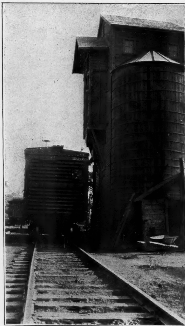
Storage Silo at Middle Granville Railroad Station
